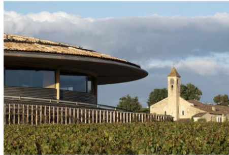
The building has been partially embedded into the ground to minimise its visual impact on the Unesco-protected landscapes
