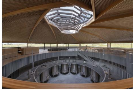
Spanning 40m, the building's dome-shaped roof features a central 6m-wide skylight that allows natural light to flood into the building, where a circular atrium lets visitors look down onto the wine production and storage spaces
