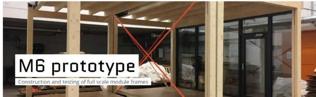
The first two M6 modules have been assembled in Harmet's Kumna factory and transported to the Estonian University of Life Sciences in Tartu, where a glass facade system was installed on one of the modules.
