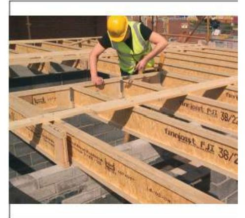
Figure 2.94. Wooden I-joist with LVL flanges.
